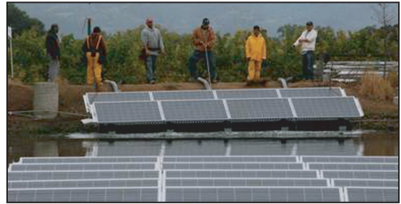
The Floatovoltaic system floats solar panels on pontoons that sit on the surface of a pond. GREG ALLEN
